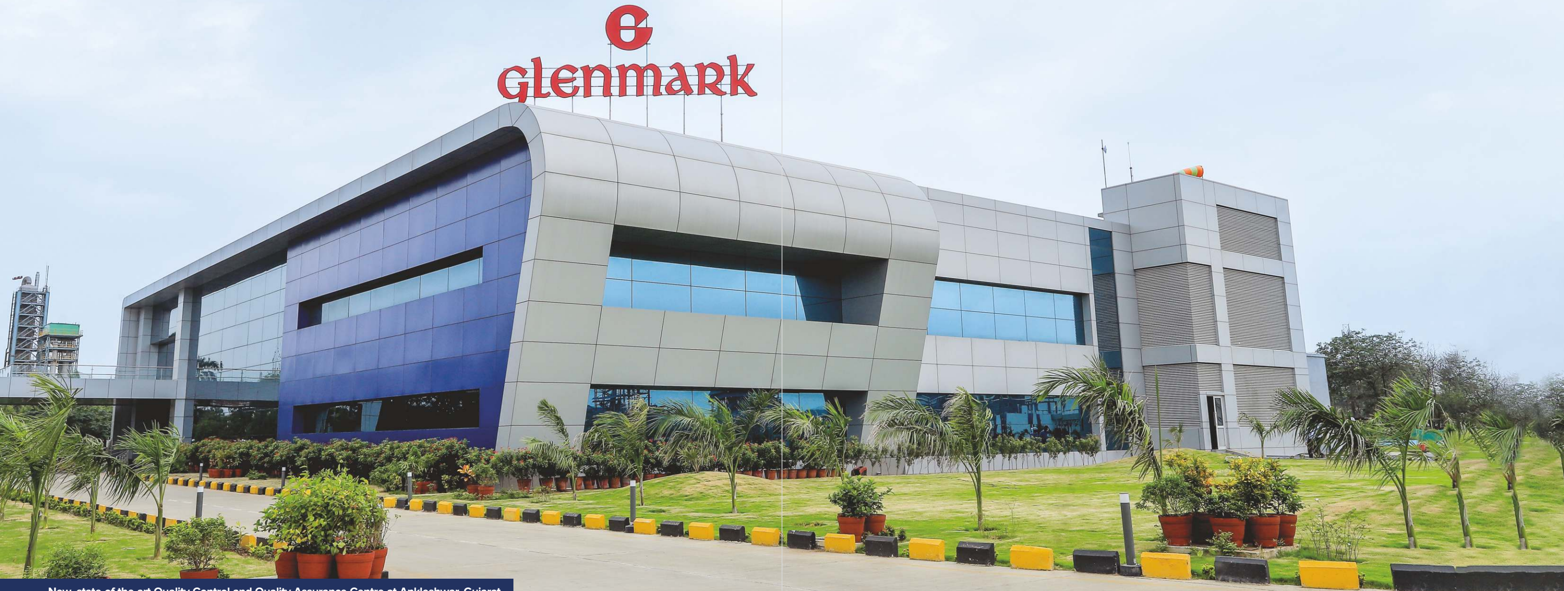
New, state-of-the-art Quality Control and Quality Assurance Centre at Ankleshwar, Gujarat.
