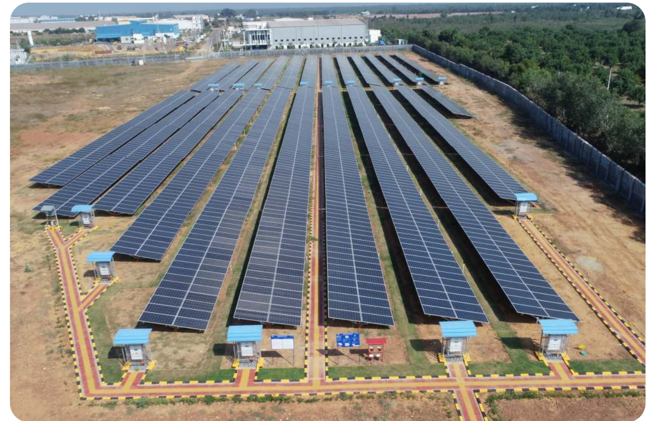
Industrial Site Sri City, Andhra Pradesh
