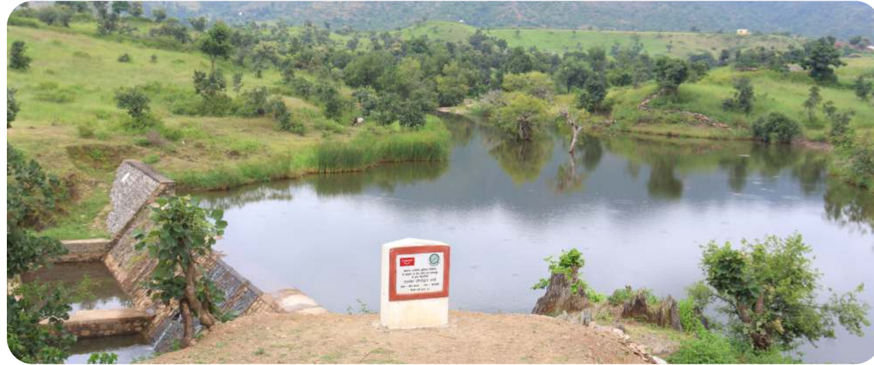
Anicut Restoration, Kaliwas Village, Rajasthan
