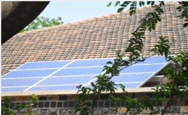
3 kW Solar PV System running at Bodhi Vriksha (MMDC), Nashik
