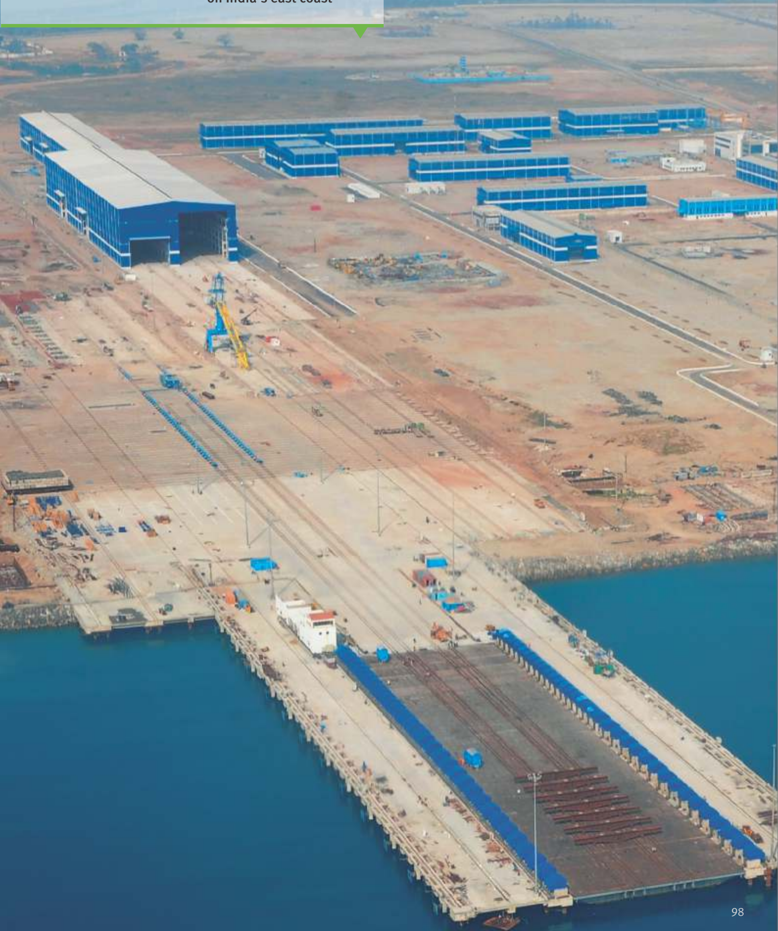
L&T's shipyard at Kattupalli, near Chennai on India's east coast
