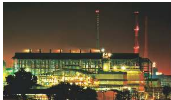
Complete Industrial Electrification solutions by L&T at Hindustan Zinc Ltd., Chanderiya, Rajasthan
