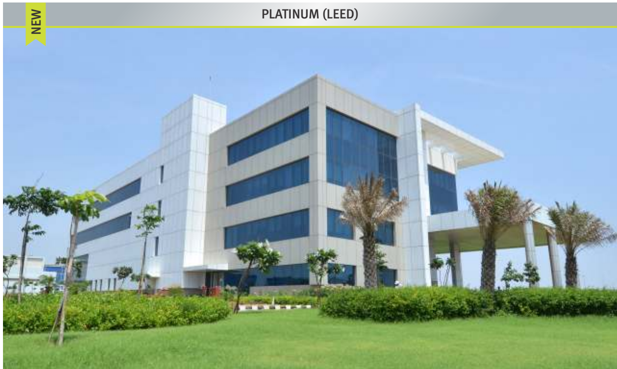
Administrative Building, Kattupalli
