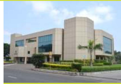
SBU Block (2 nd floor), Hazira
