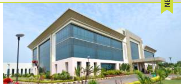
Administrative Building, Vadodara
