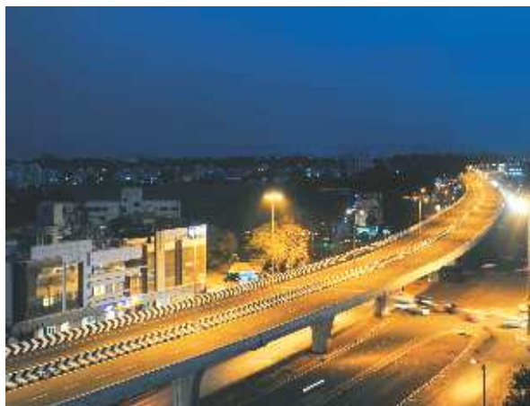
Elevated road corridor at Nashik, near Mumbai
