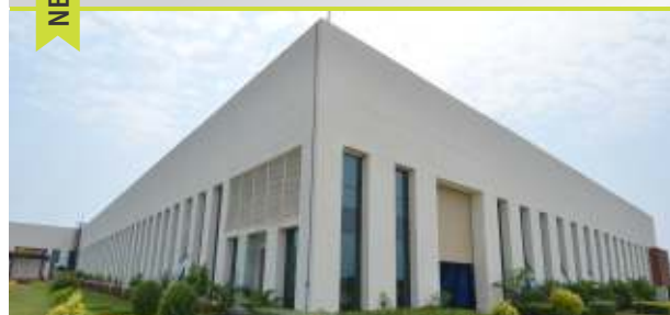
Green Factory, Vadodara
