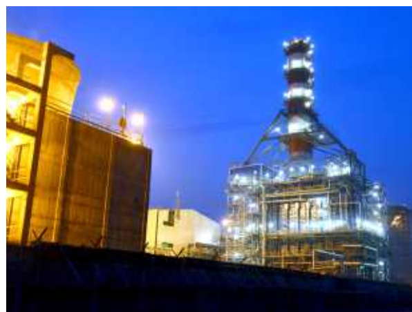
Power Plant at Dhuvaran, Gujarat
