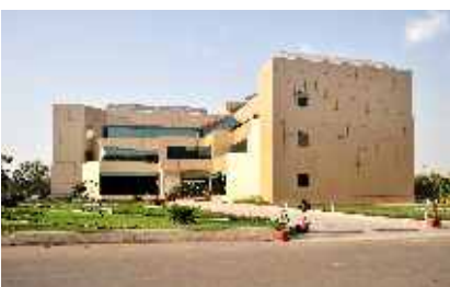
Administrative Building, LTSSHF, Hazira
