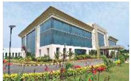
Administrative Building, Vadodara
