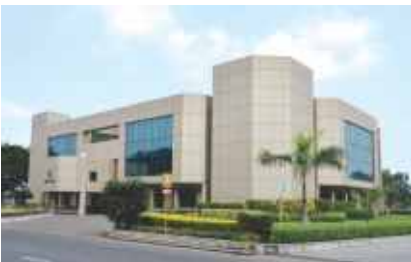
SBU Block (2nd floor), Hazira
